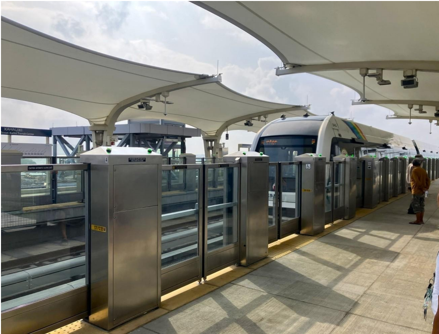
Platform screen doors (PSD) are at all Skyline stations, as seen here at the Kahauiki (Kalihi Transit Center) station, the current eastern terminus of the line.
