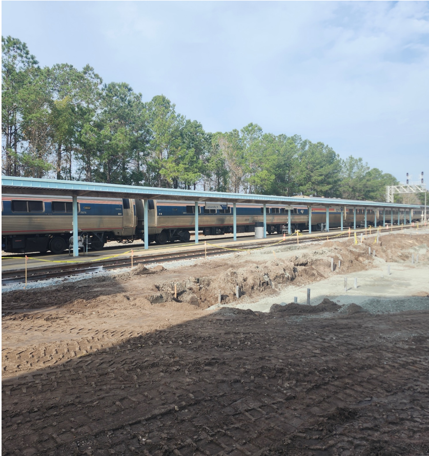
Renovations at Amtrak's Jacksonville station are underway.
