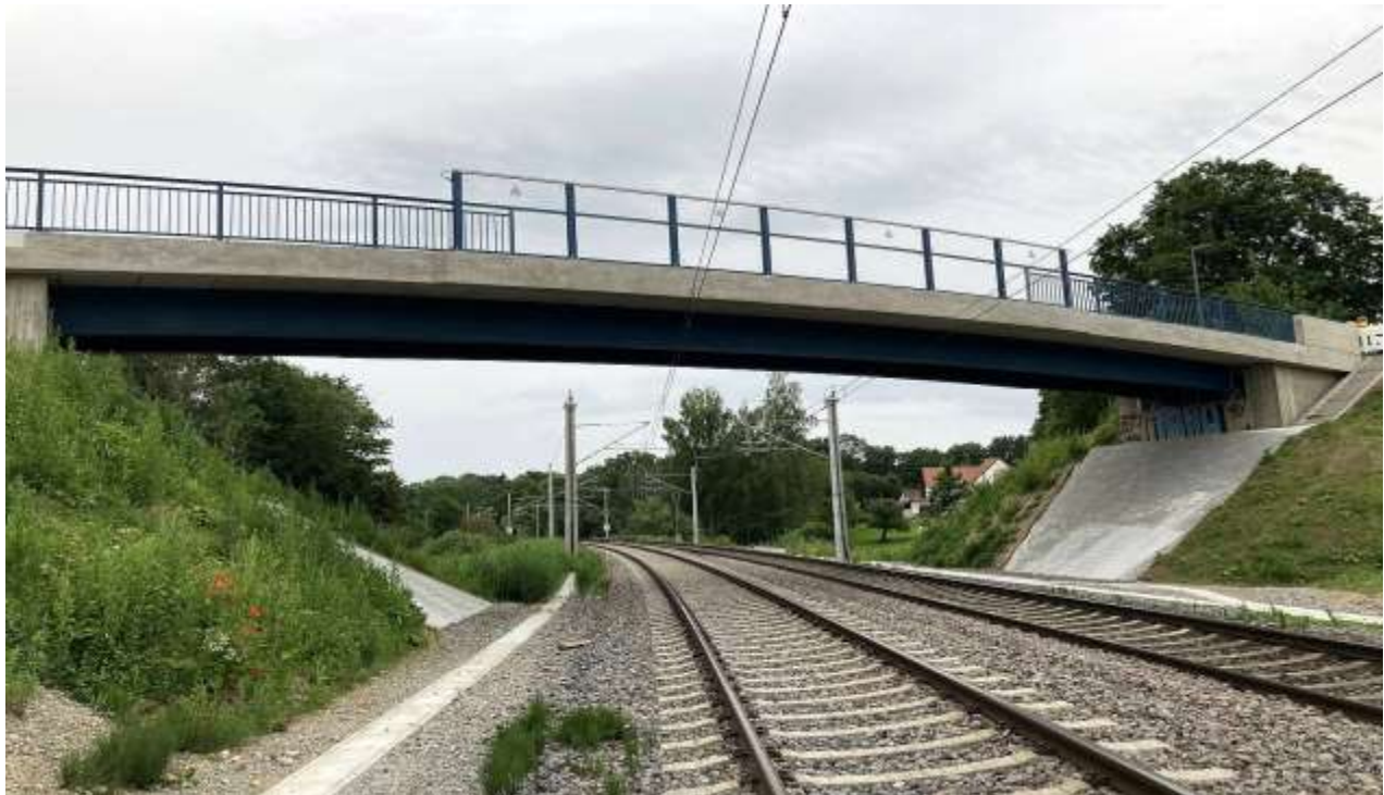
Bridge over historic rail line - view of the "Südbahn" just south of Aulendorf in July 2021. The new electrification infrastructure is complete at this point, but not yet energized. A new replacement bridge, one of two which were not paid for by the electrification project, is nearly finished and has already been attacked by local graffiti artists. The funds for this new replacement bridge (the original one was demolished to clear the way for the electrification catenary) were located in a special state infrastructure fund for repair and rebuilding local streets and roads not designated as federal or state roads within this German state.
